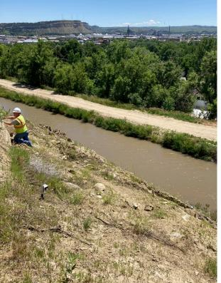
Triaxial Tiltmeters were installed on stakes, to assess ground stability, as well as directly onto large boulders
